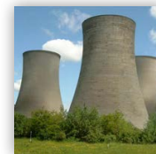
Utility, Safety, & Facility Systems
